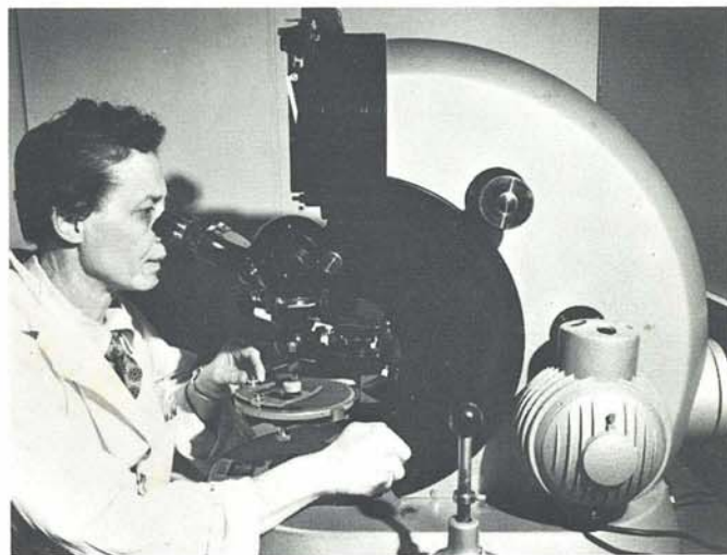
Mrs. Doris Cheever examining a ceramic polished section at the Zeiss Ultraphot II Metallograph.
