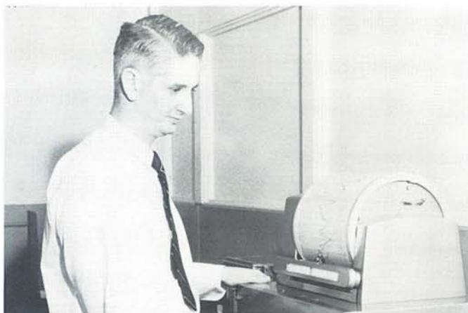
MR. GEORGE MAC BRIDE, Engineer, in the chemical development lab is running a sample of trichloroethylene for impurities on the Perkin-Elmer 421 grating infrared spectrophotometer.
