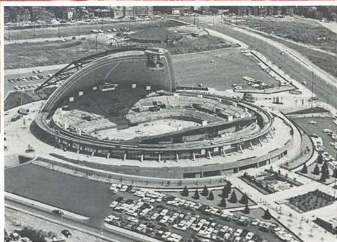
UNBELIEVABLE UMBRELLA magnificently reposes in Pittsburgh's front yard to add interest for 1962 conferees. This $22 million, giant steel umbrella covers the new Public Auditorium -- destined to become one of the great meeting places of the world. At the touch of a button, the steel "umbrella" which forms the roof will "fold up" to provide a huge outdoor arena accommodating up to 13,000 persons.
